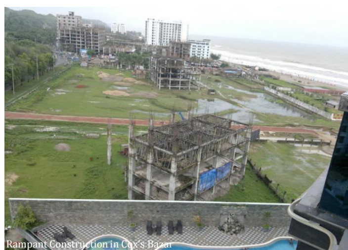
Rampant Construction in Cox's Bazar
