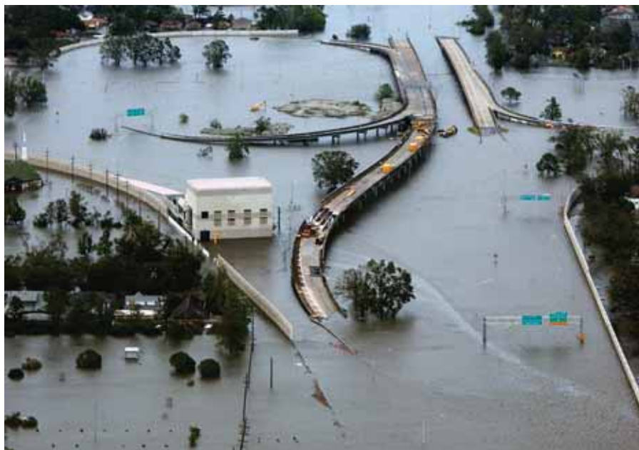
New Orleans following Hurricane Katrina, looking towards Lake Pontchartrain
