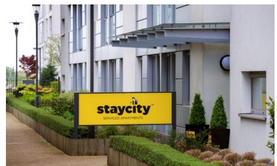
Above: Staycity in Hayes, London – acquired in March 2016 by Schroder UK Real Estate Fund (SREF) for £32.4m, 5.5% initial yield.
